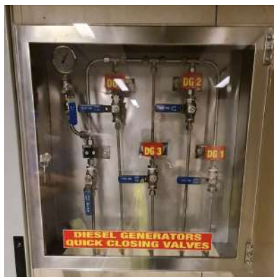
Complete Fuel Flow meters / quick closing valves installation (including compressed air plant and electrical wiring)
