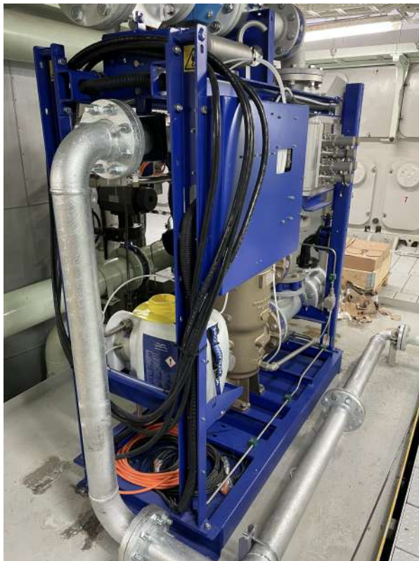
Complete installation of Ballast Water Treatment Systems
